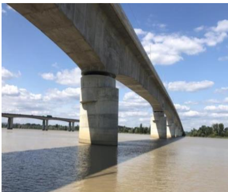
Figure 3: LGV Sud Europe Atlantique bridge on the Dordogne river near Bordeaux. Source: Artelia
