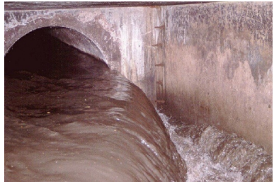
Storm water overflow sewer
