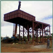
Hoppers and bunkers
